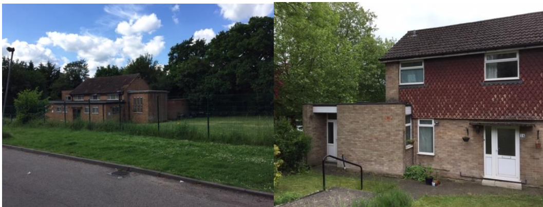
(Left) The former church of St Francis
